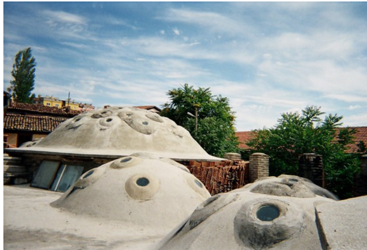
Photo 2: HAMMAM, Ankara, Turkey / Photo interview 03: Roof of Shengül Hammam [3]
