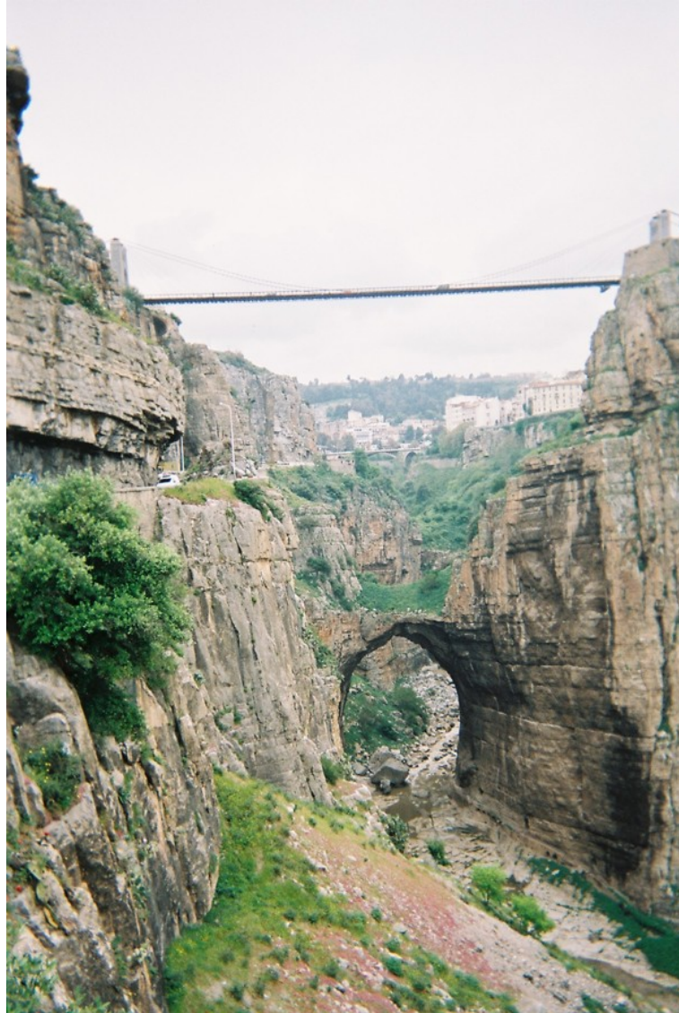
Photo 8: HAMMAM, Constantine, Algeria / Photo interview 01: Sidi M'Cid Bridge [34]
